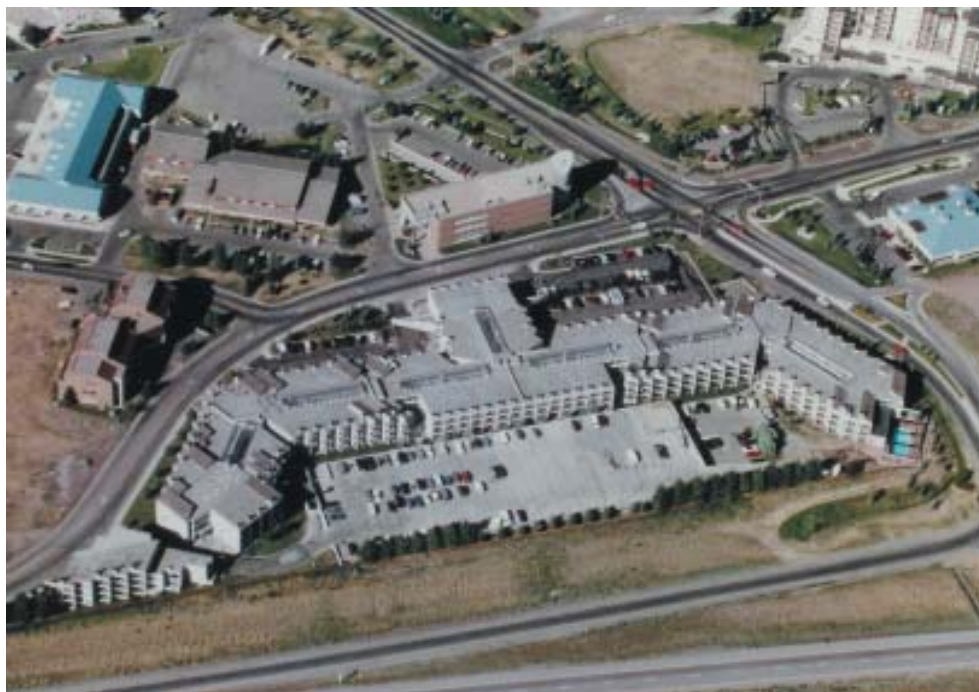
Note the scarcity of buildings surrounding the Lodge. You might be able to recognize (clockwise from left of the Lodge): Buck Creek Plaza, the Annex, Benchmark Shopping Center, Boat Building, Lodge at Avon and 1ST-Bank. That's I-70 running below the Lodge, and the top of the picture is pointing south. Notice the desolation and lack of cars on I-70!
